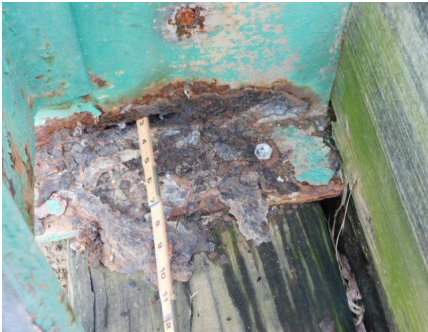
SPAN 1 HOLE IN STEEL I BEAM
